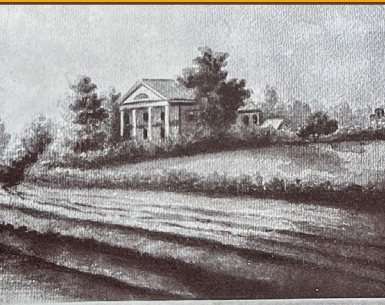
Illustration of Arlington Plantation alongside the Mississippi River; Ripley, E. (1912, 1975). Social life in old New Orleans. Arno Press.
